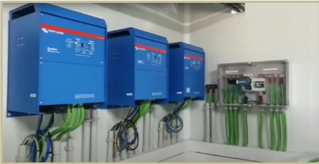
Image 3: Inverters and voltage and voltage regulators
