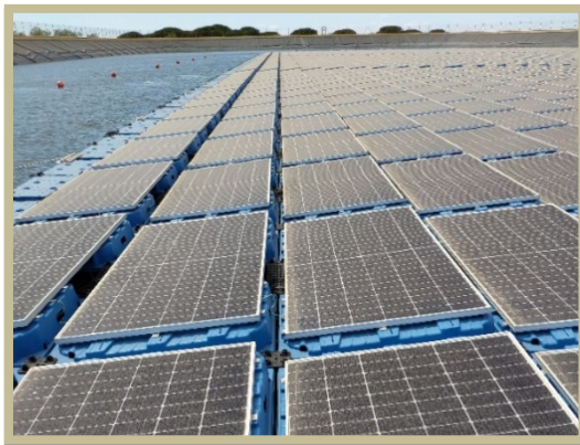
Image 2: Detail view of floating photovoltaic installation
