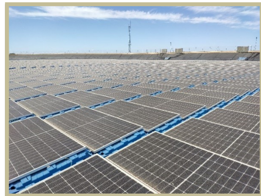
Image 2: Detail view of floating photovoltaic installation
